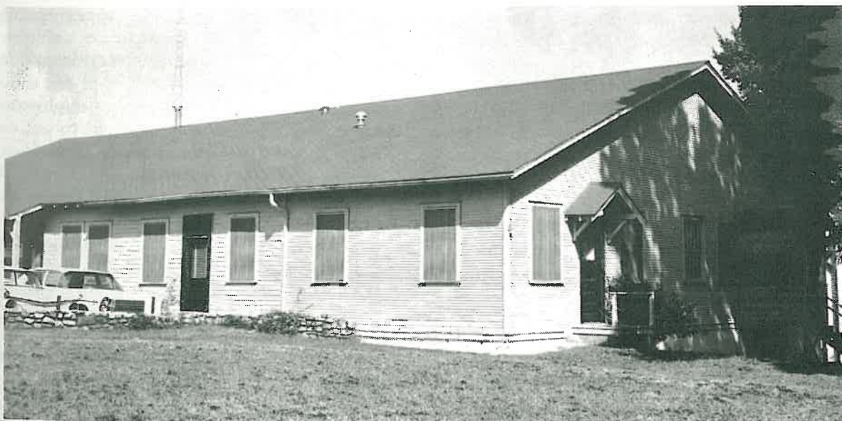
The original offices of the Highway Department were housed in the basement of the State Capitol. In 1927, the wooden structure here was built for use by the engineers. Later on, another section was added to it. From that time until the move, some phase or phases of AHD operation had used the old facilities. In 1938, the WPA built the four-story building just vacated. We've come a long way. (More pictures on page 13.)
