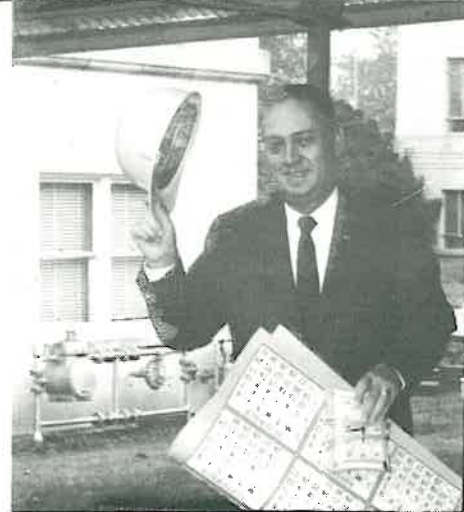
At top, Mr. Hicks makes a last minute check for anything left behind. Below, Mr. Goodman tips his hard hat in farwell to the old building. The windows of Mr. Goodman's old office are in the background.
